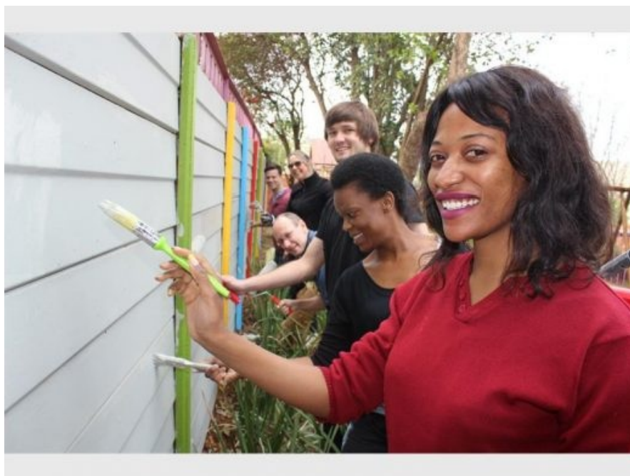
Kuka Mofu and her colleagues repaint the school's wall. Photos: Siso Naile.
